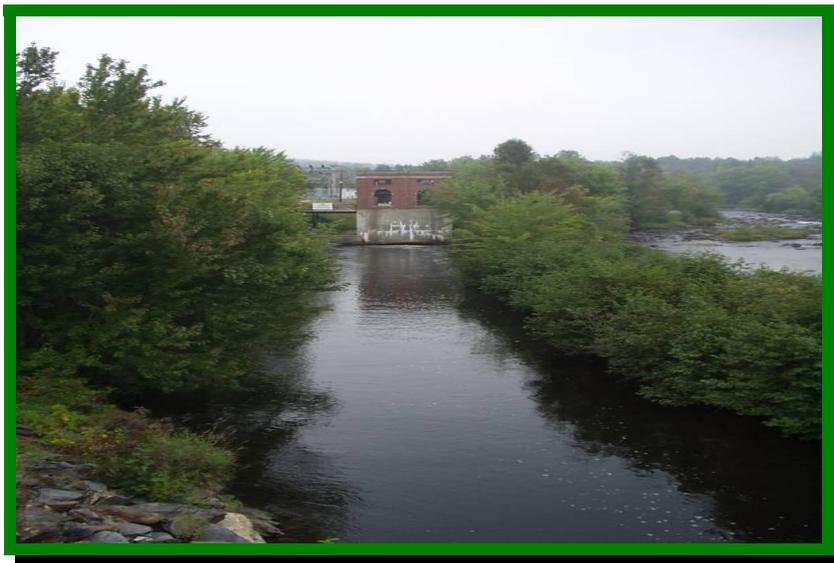
The estimated average generating head is 35 feet. The estimated average annual generation is 7,300,000 kilowatt-hours. The impoundment is approximately 4,000 feet long with a surface area of about 20 acres and a gross storage capacity of approximately 200 acre feet.
